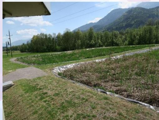
Sludge drying reed bed scheme (left) and live (right) (source: Limnos)
